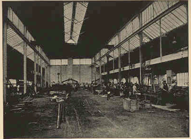
Engineers' and Smiths' Shop.
