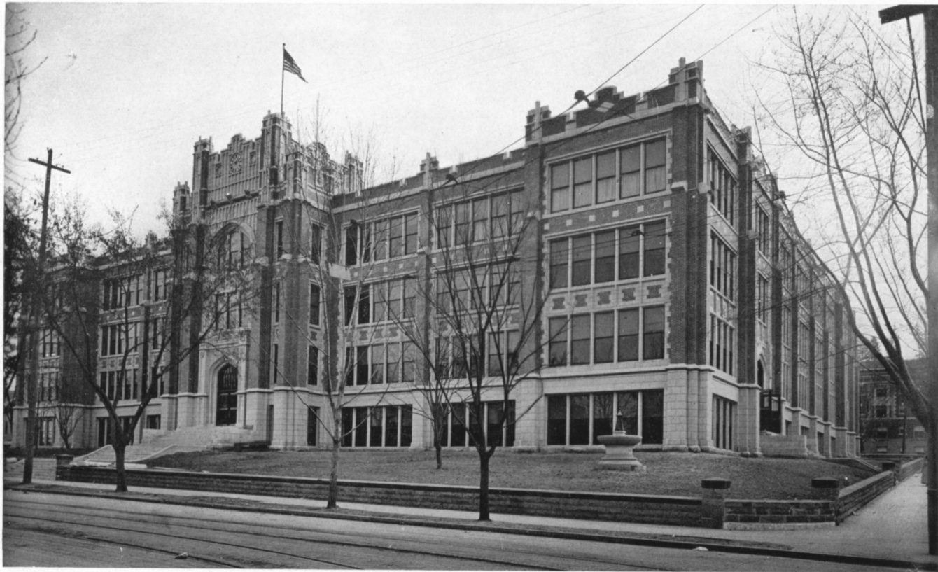
LEWIS & CLARK HIGH SCHOOL, SPOKANE, WASH. All the School Buildings of Spokane Are Equipped with Mason Safety Tread.
