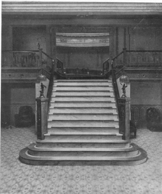
ROGERS HOTEL, MINNEAPOLIS, MINN. Marble Stairway, Brass (Delta Metal) Base, Mason Safety Tread Used
