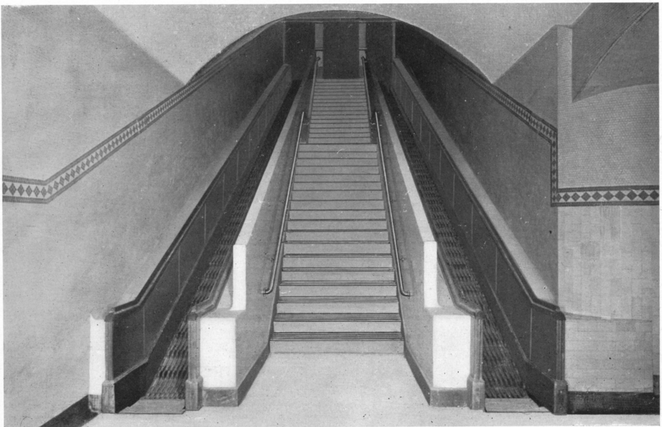
MASON SAFETY TREAD, STEEL AND CARBORUNDUM, SET IN CONCRETE STAIRS State Street Station, Boston, Mass., Washington Street Tunnel
