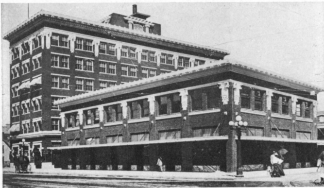
TERMINAL AND ARCADE BUILDINGS, OKLAHOMA CITY, OKLA.
