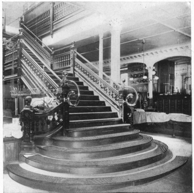
CURVED STRIPS OF MASON SAFETY TREAD ON WOOD STAIRS.
