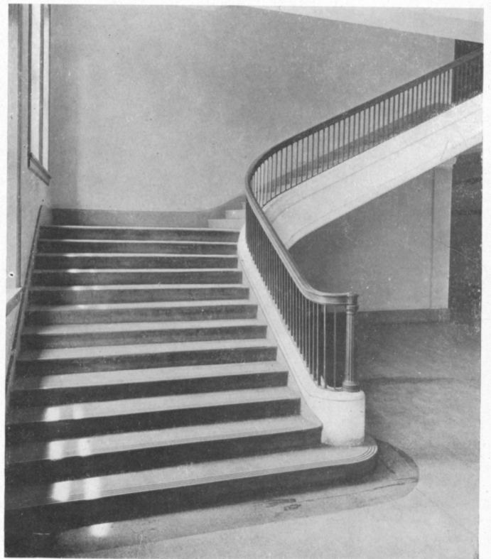
McKINLEY MANUAL TRAINING SCHOOL, WASHINGTON, D. C. Main Stairway, Treads and Risers \frac{1}{2} Inch Thick, Karbolith with Lead Filled Mason Safety Tread on Front Edge
