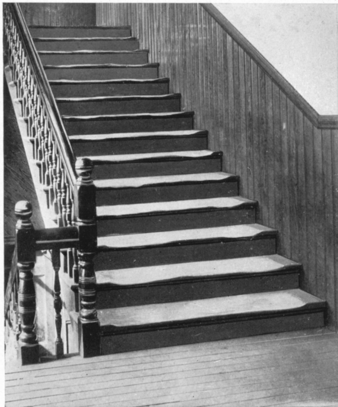
Before Repairing MASON SAFETY TREAD, KARBOLITH AND CORK COMPOSITION REPAIR WORK ON WOODEN STAIRS AT THE ST. JOSEPH'S CATHOLIC COLLEGE, LOWELL, MASS. After Repairing
