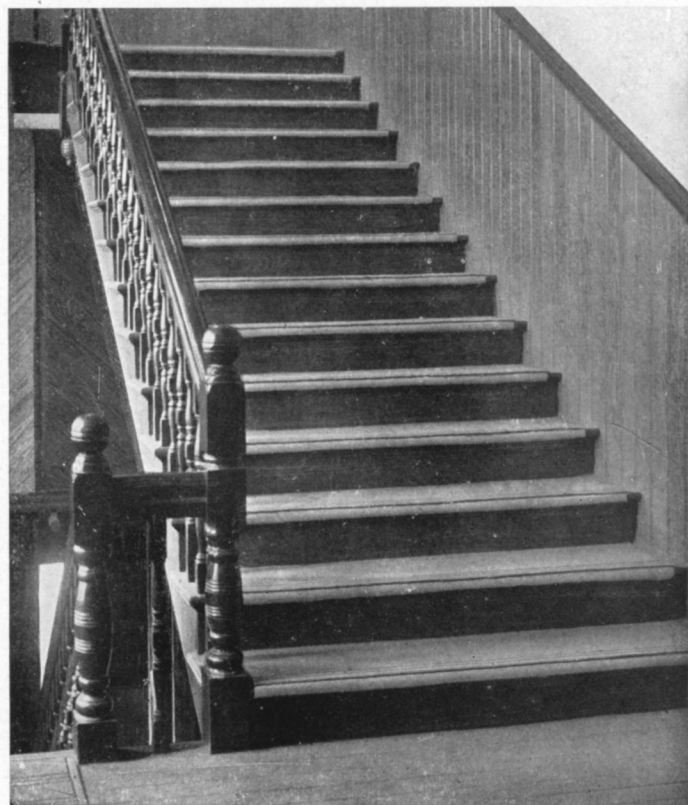
Before Repairing MASON SAFETY TREAD, KARBOLITH AND CORK COMPOSITION REPAIR WORK ON WOODEN STAIRS AT THE ST. JOSEPH'S CATHOLIC COLLEGE, LOWELL, MASS. After Repairing
