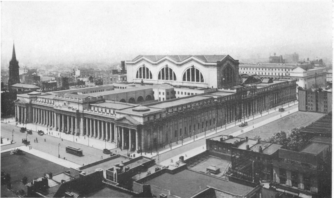
PENNSYLVANIA RAILROAD TERMINAL AT NEW YORK CITY Mason Safety Tread Used
