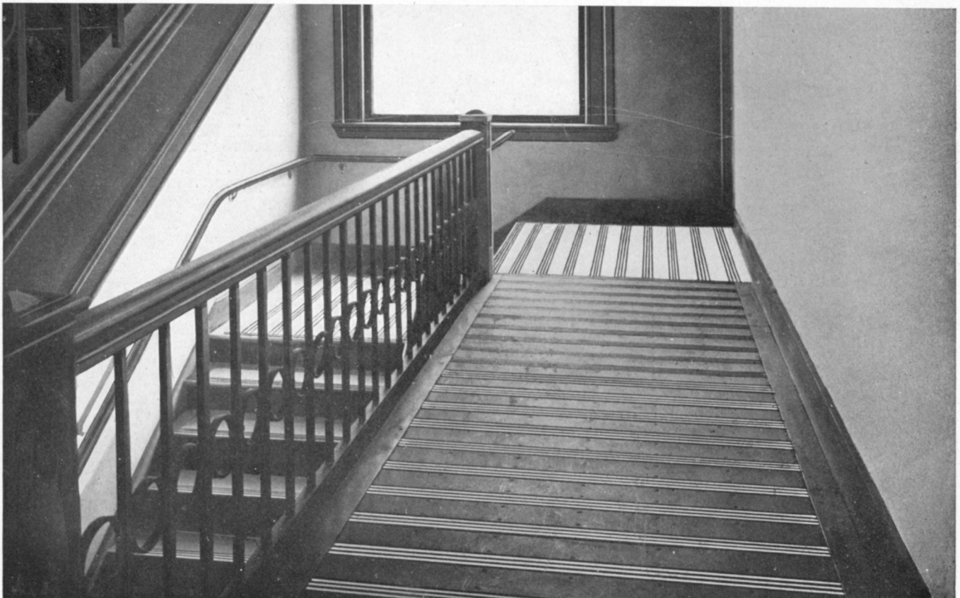
MASON SAFETY TREAD AND CORK COMPOSITION ON IRON STAIRS AND LANDINGS Houghton & Dutton Co., Department Store, Boston, Mass.
